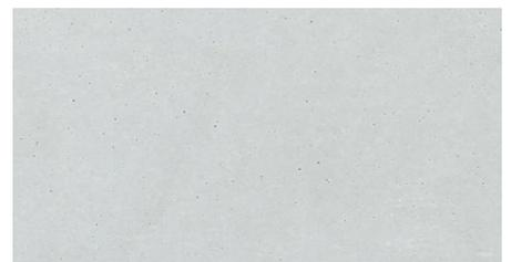
Small air bubbles and porosity are possible: data sheet on exposed concrete 06/2015 (Publ.:BDZ/DBV)
